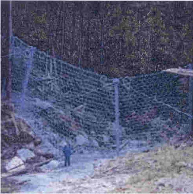
Figure 7. Geobrug UX debris flow barrier (Source: Geobrug Fatzer, AG).
