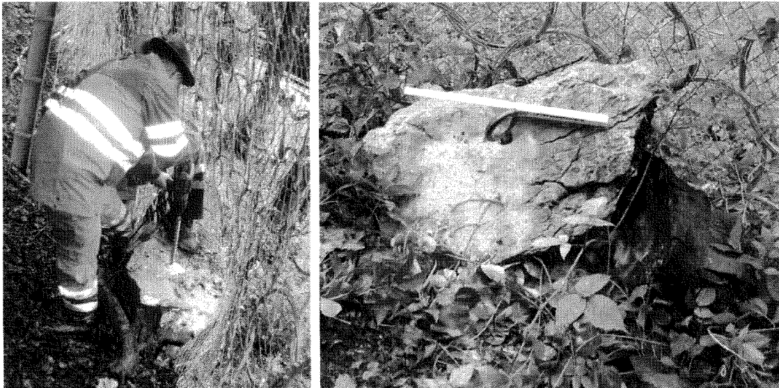
Figure 4 Providing the block with towing hooks
